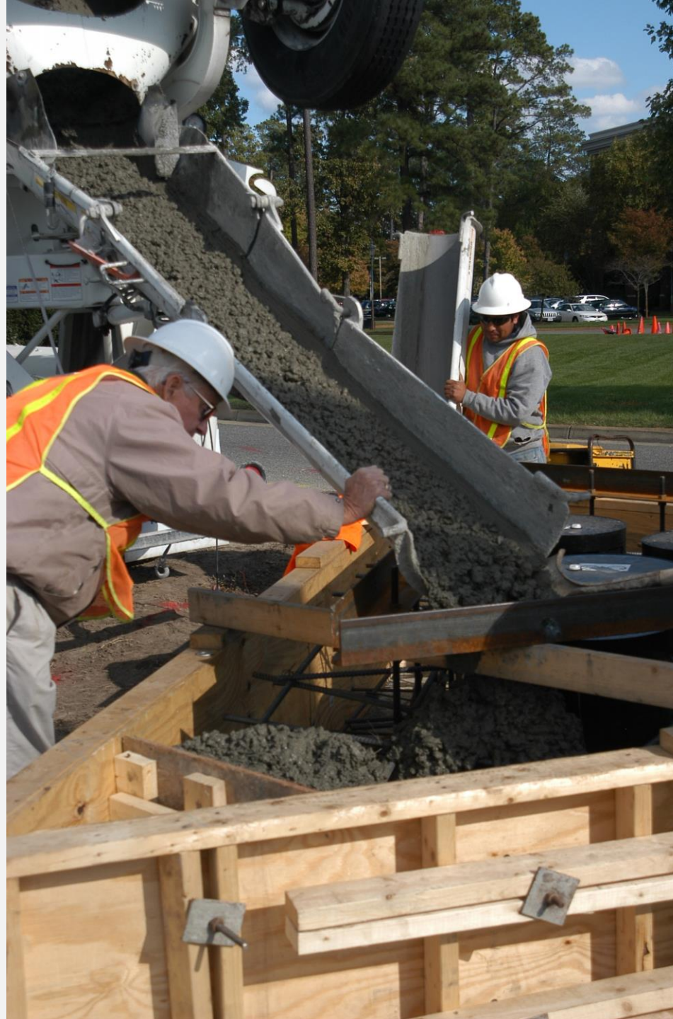
Pouring concrete for the base of Izar .
